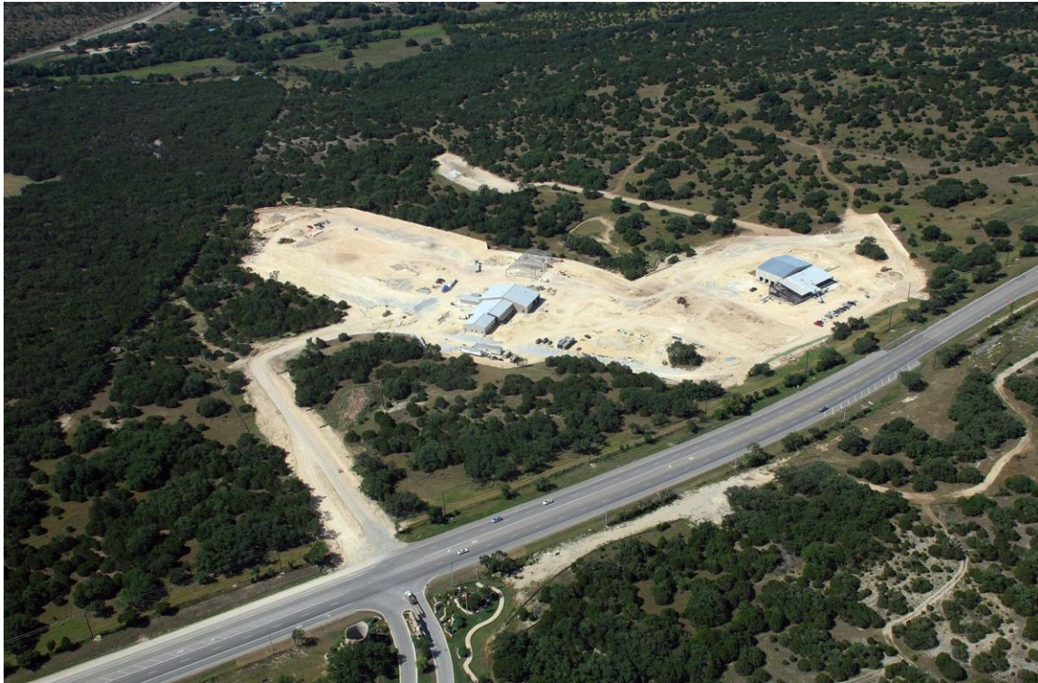
Transportation Center / Distribution Center site photo taken 8/5/10
