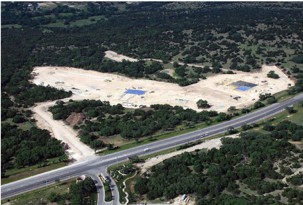
Transportation Center / Distribution Center site photo taken 5/6/10
