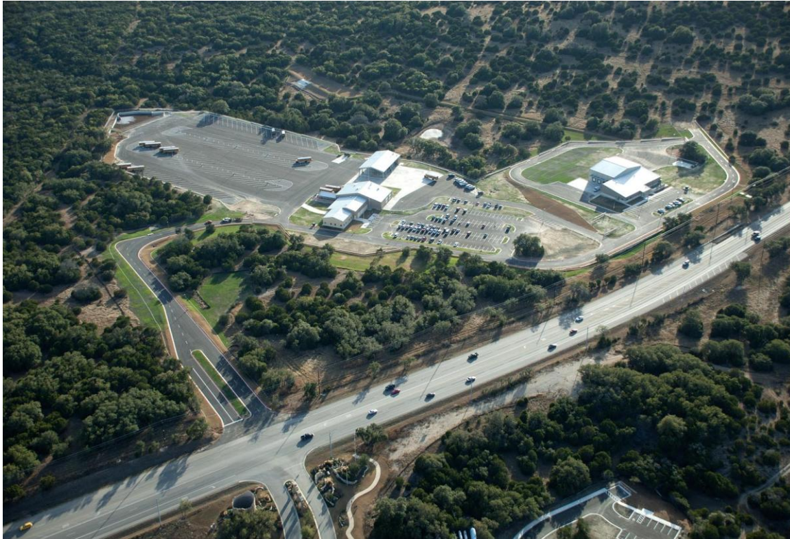
Transportation Center / Distribution Center site photo taken 1/7/11
