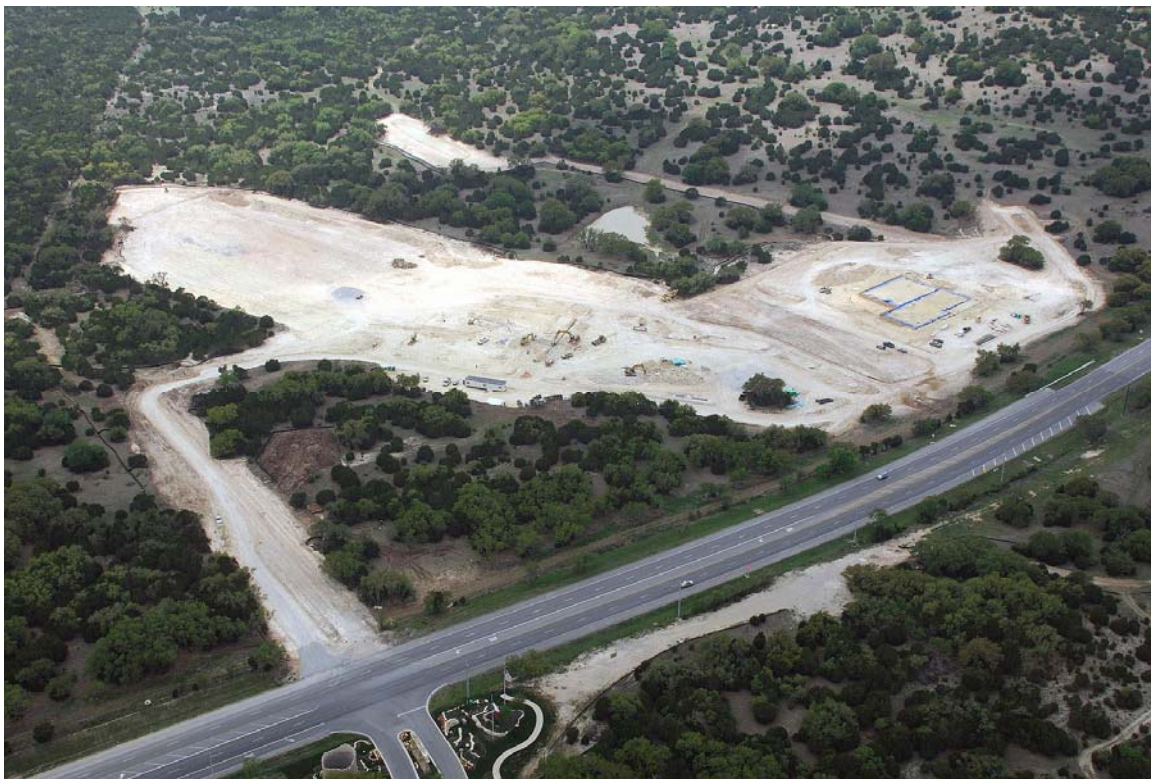
Transportation Center / Distribution Center site photo taken 4/6/10
